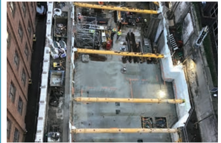
Aerial view of the construction site, with application of PREPRUFE® 120S
