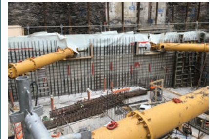
Rebar installed against the PREPRUFE® 120S membrane
